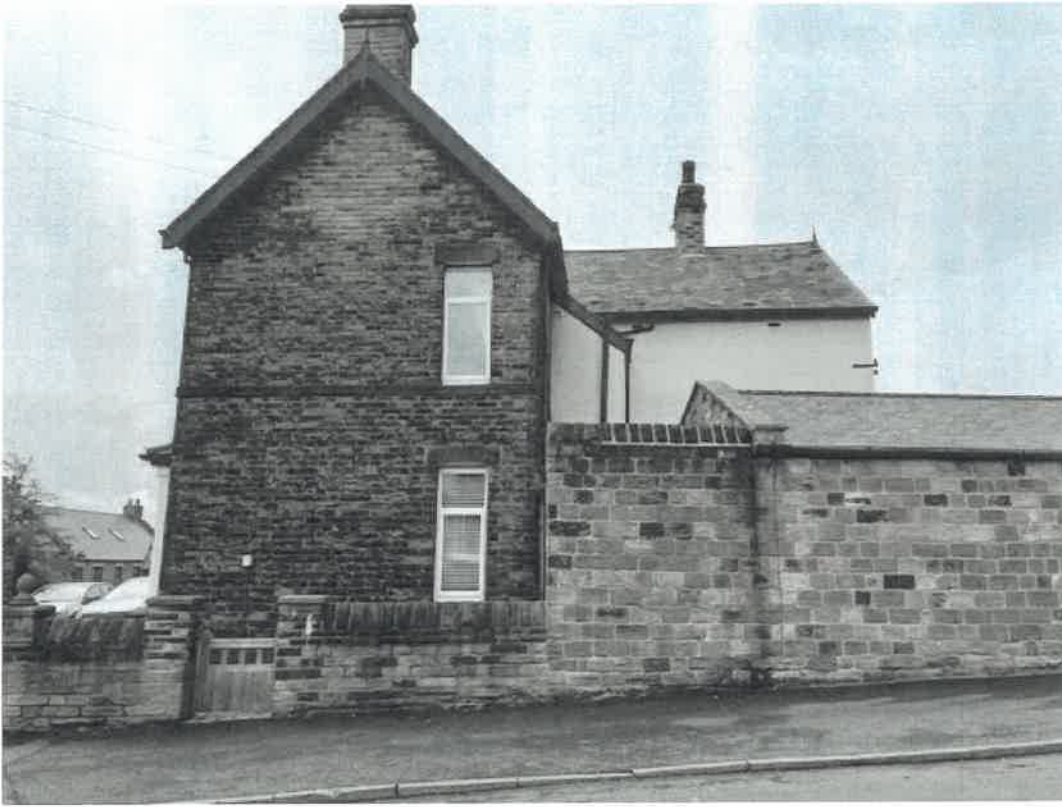
VIEW FROM NORTH & CLAREL STREET
