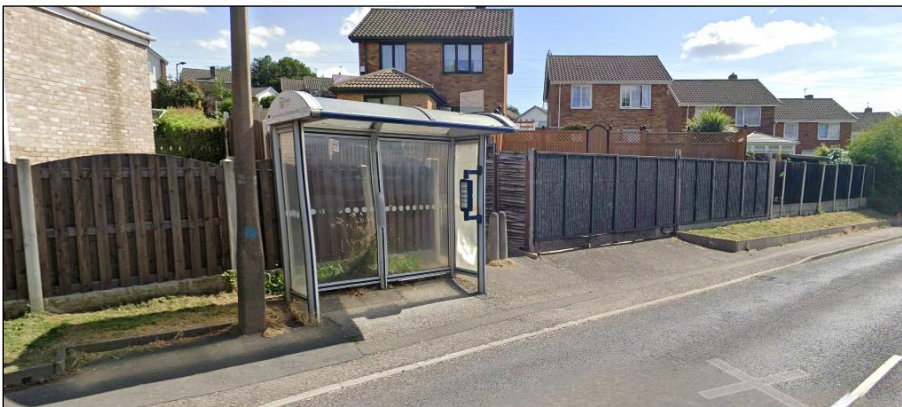
Figure 6: 55340 (outbound)- 2-bay P1 shelter (Image source: Google, July 2025)
