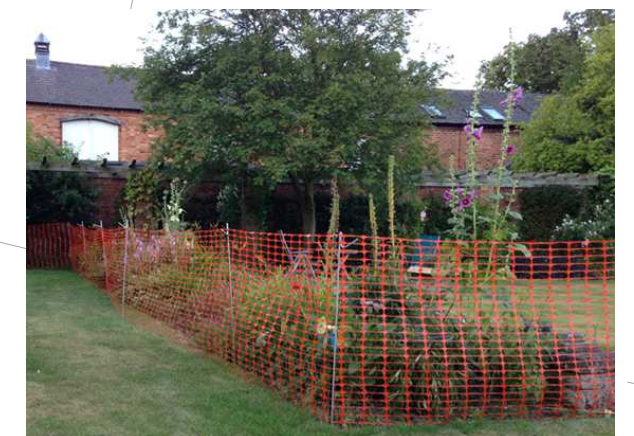
Inset 2: Plastic Mesh Tree Protection Fencing
