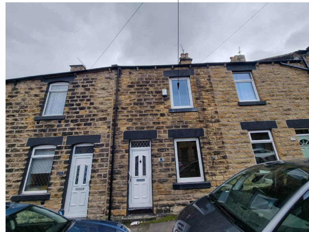
Replacement modern windows, stone head and cills
