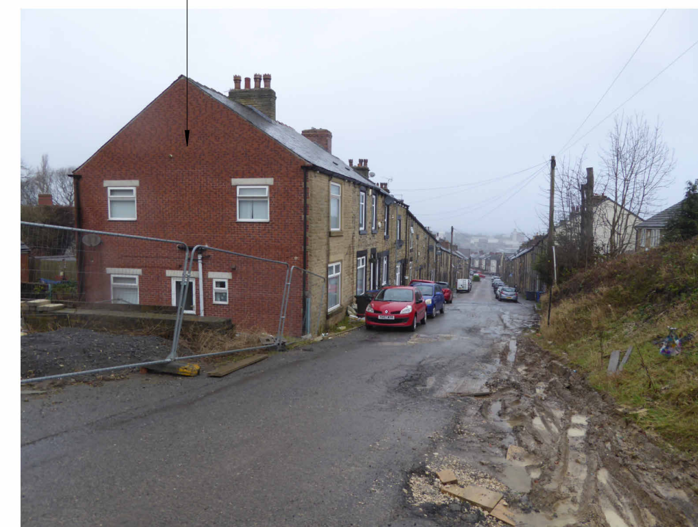
52 Tower street set back from building line of terraced houses. Modern window configurations. Stone facing materials, no stone cills or lintels
