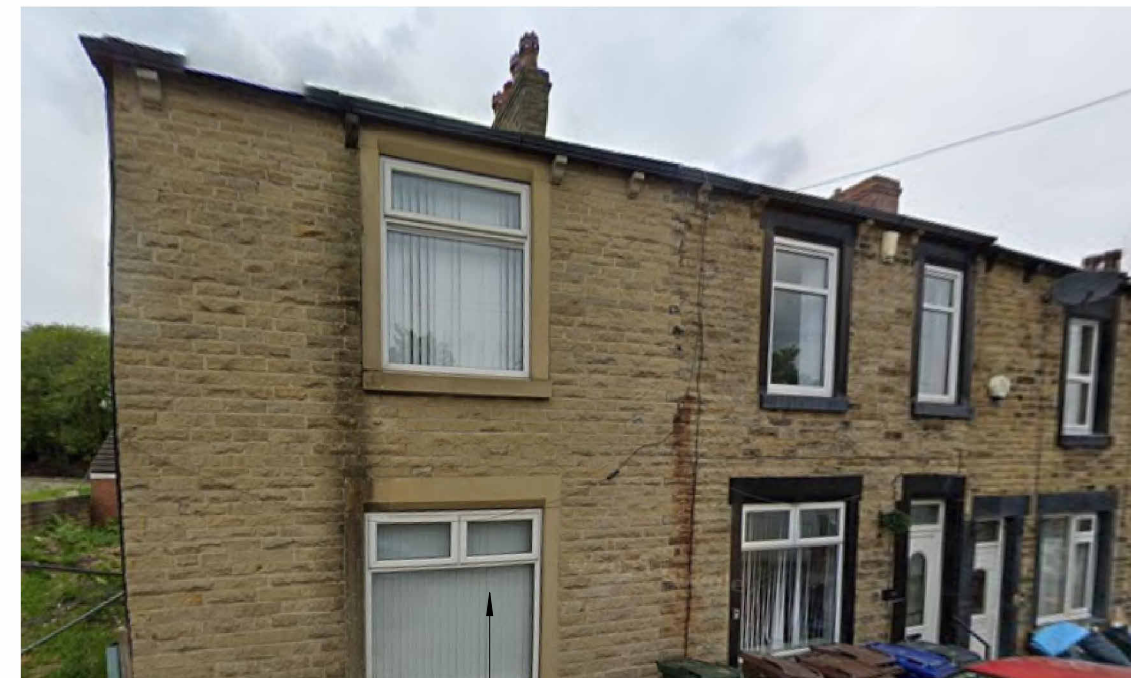
No 63 opposite the proposed dwelling with side extension to form double fronted dwelling, stone window surrounds.
