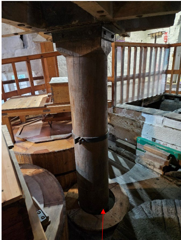
Entrance point of shaft from ground to first floor Length: 5800mm Width: 800mm at widest point,
