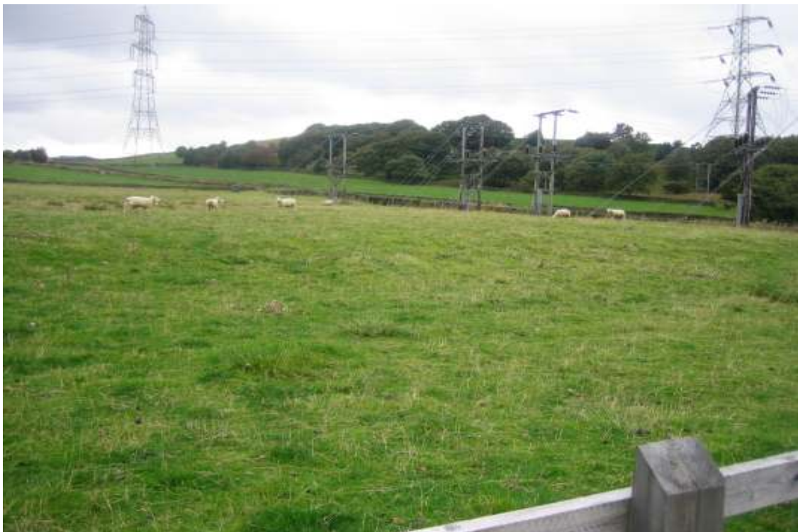
View on Front of Existing Tofts Lane Substation looking toward Tofts Lane
