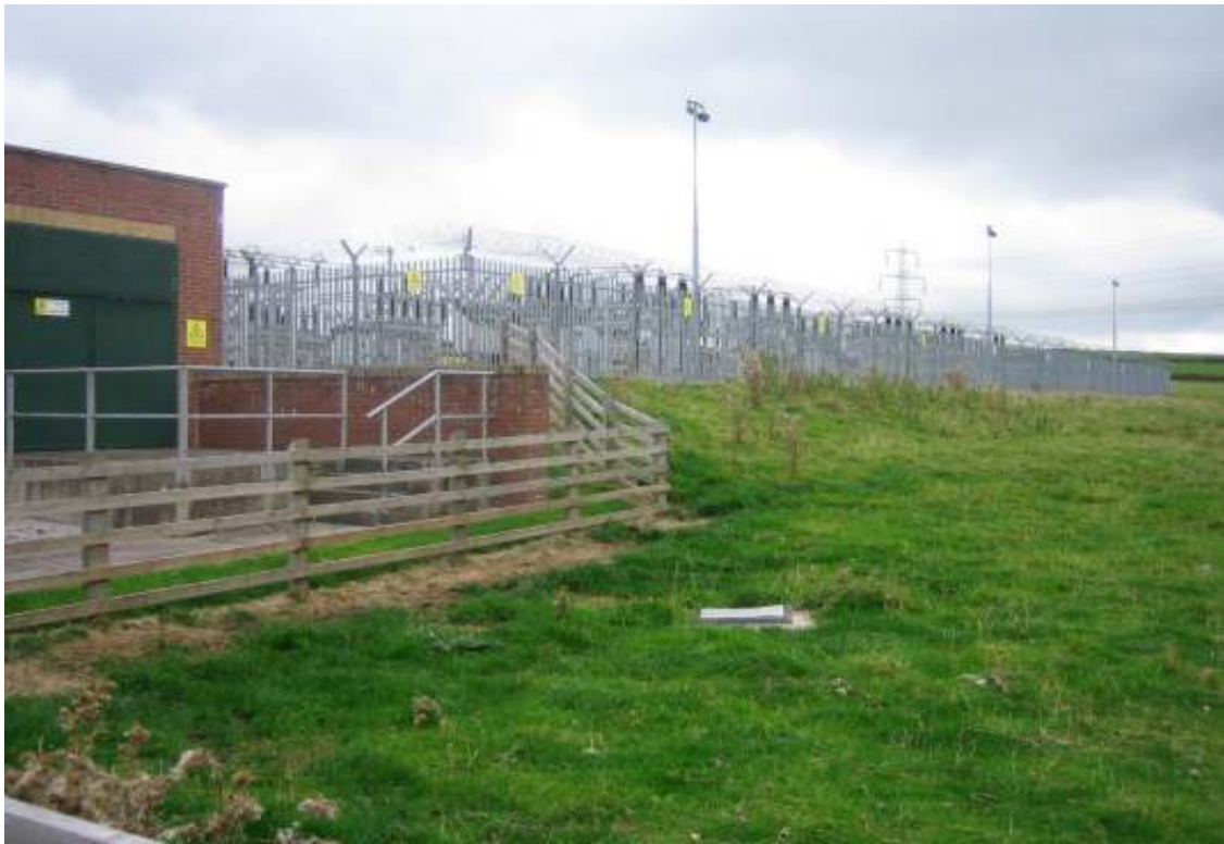
View on Front of Existing Tofts Lane Substation
