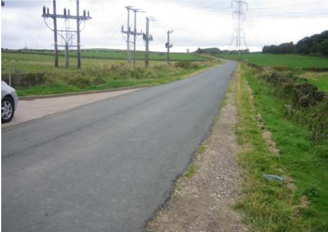
View looking North, North West on Tofts Lane.
