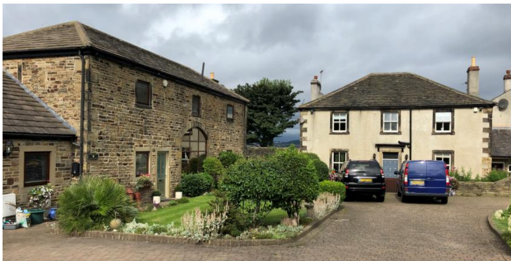
Figure 3.1: Balk Farmhouse (right) and Barn (left)
