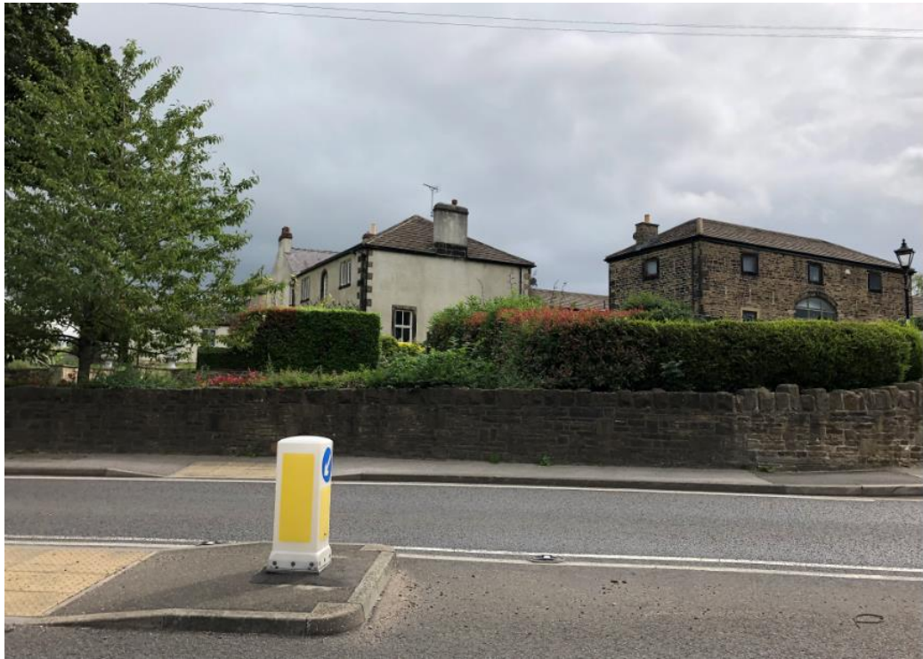
Figure 3.6: View of the Listed Building and Barn from A61 looking east
