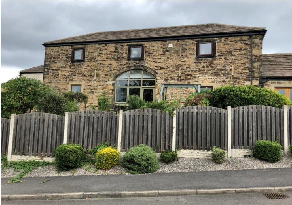
Figure 3.4: View of south elevation of the Barn from Balk Farm Court
