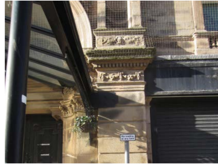
1960's replica canopy - showing door connections to the stonework
