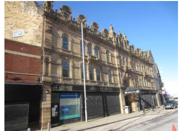
Existing Eldon Street Facade
