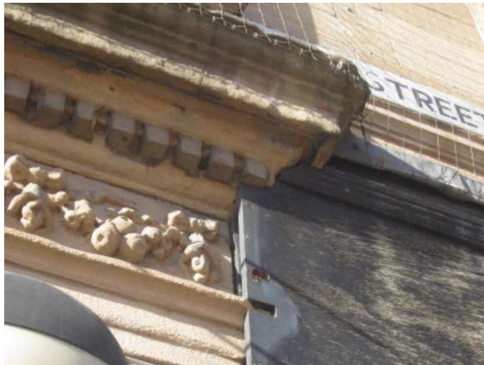
Existing signage and fascia detail
