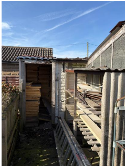
Rear of Garage
