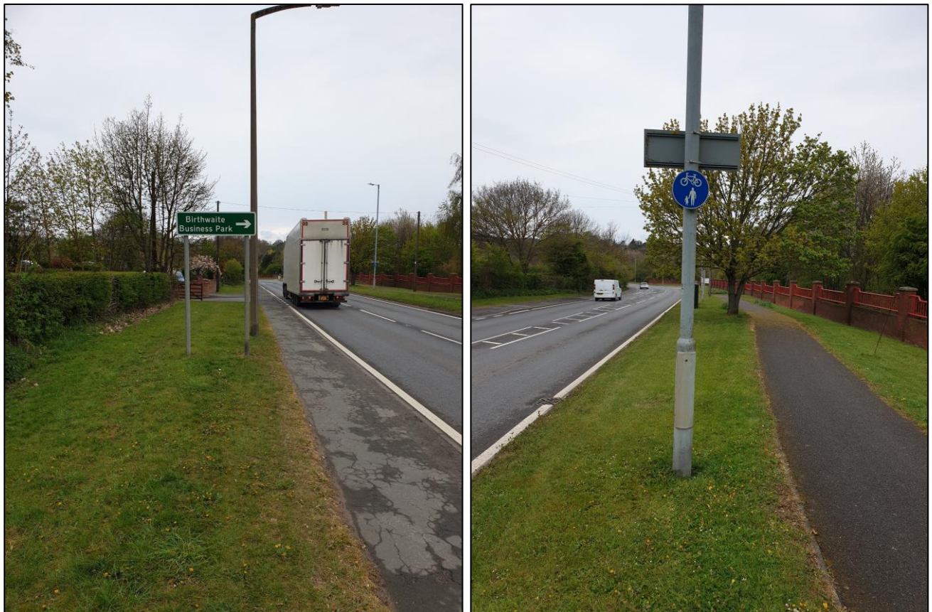
Figure 3.2 -Pedestrian Footway on Huddersfield Road in the Vicinity of the Site
