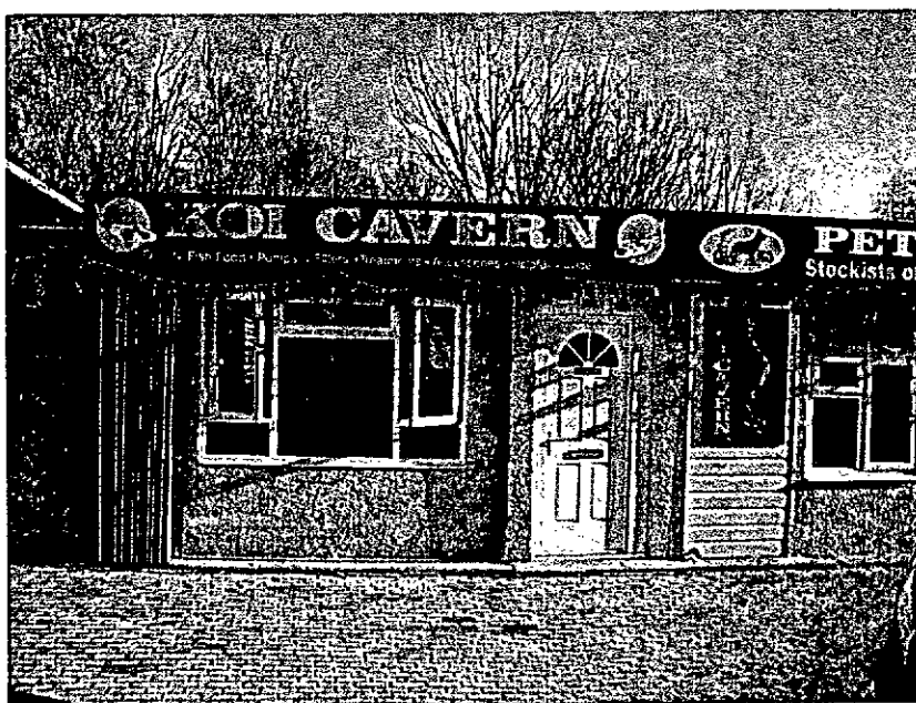
Photograph 4 Shows new pebble dash frontage to unit 2, with new infill panel and upvc window, set behind existing roller shutter door.
