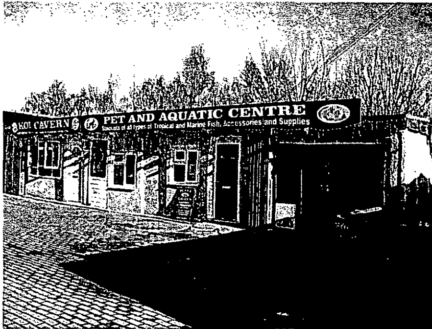
Photograph 1 Shows the site access to all the units within the complex
