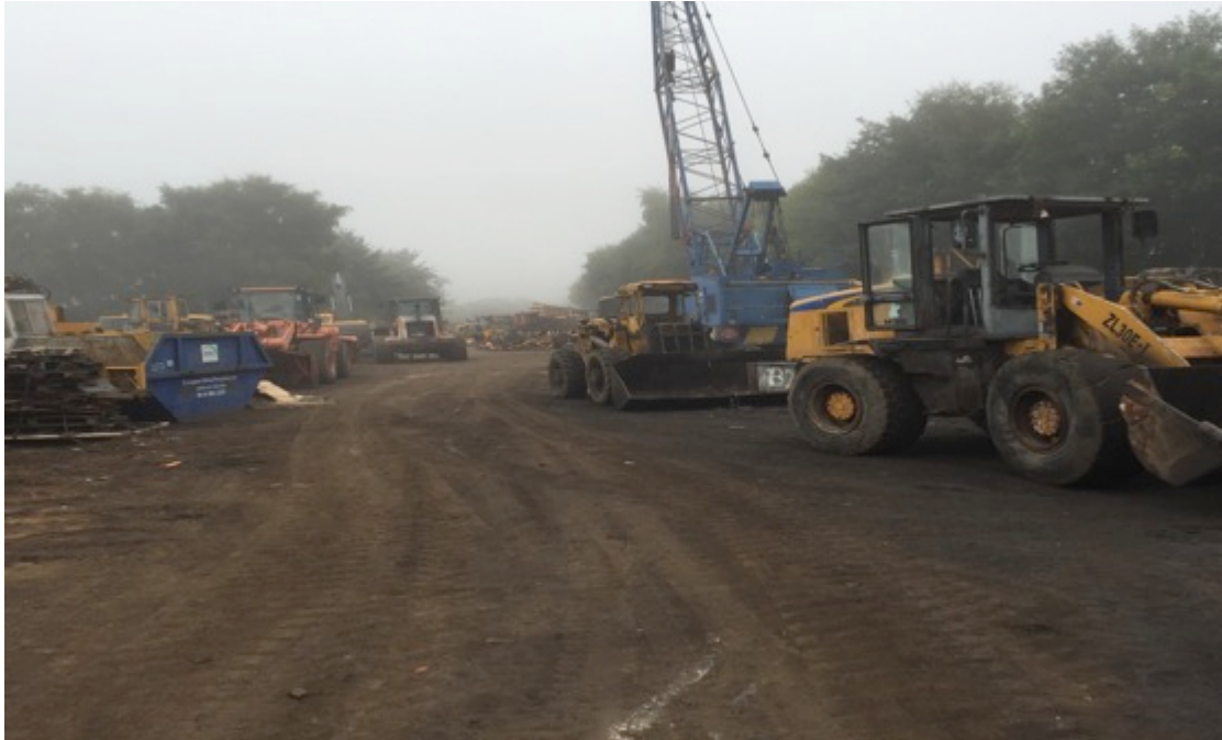
Figure 2 View looking southwards along the site. The proposed siting of workshop building is on the immediate right.
