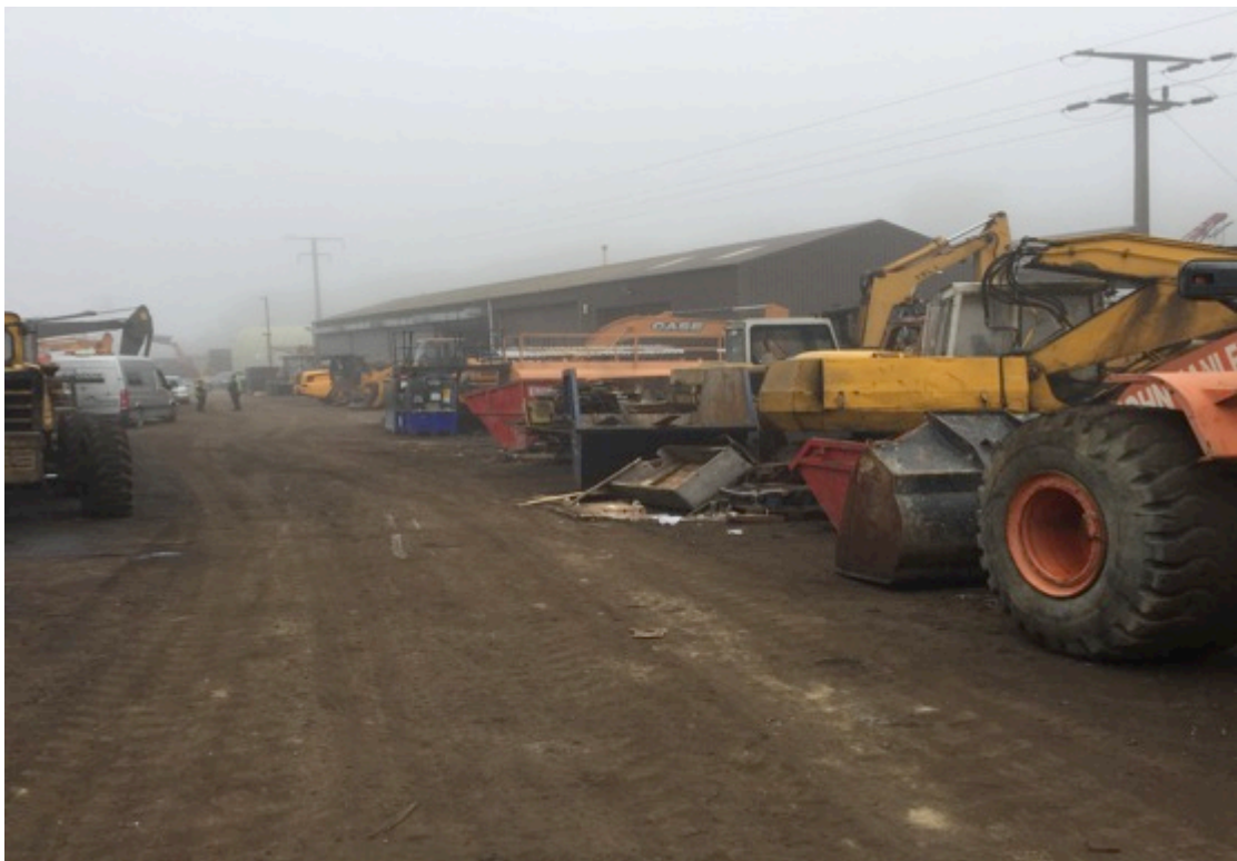
Figure 3 View looking northwards along the site showing existing workshop building
