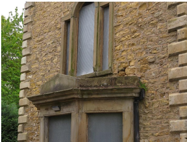
Fig 3 – Bay Window with venetian window over
