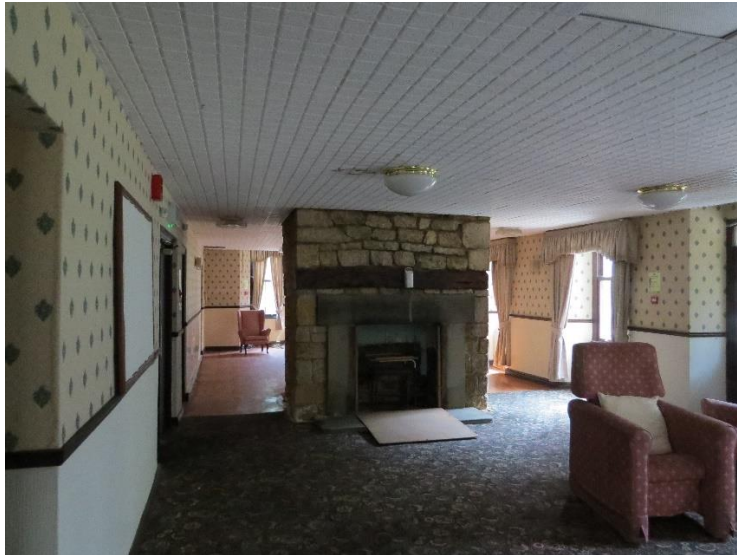
Fig 10 – Ground floor – suspended ceiling to main hall
