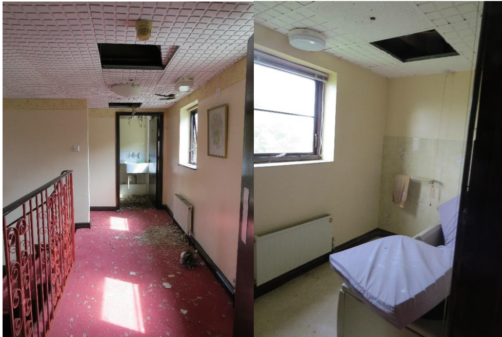
Figs 4 & 5 – Second Floor – suspended ceiling to stairs, sluice, wc and shower rooms
