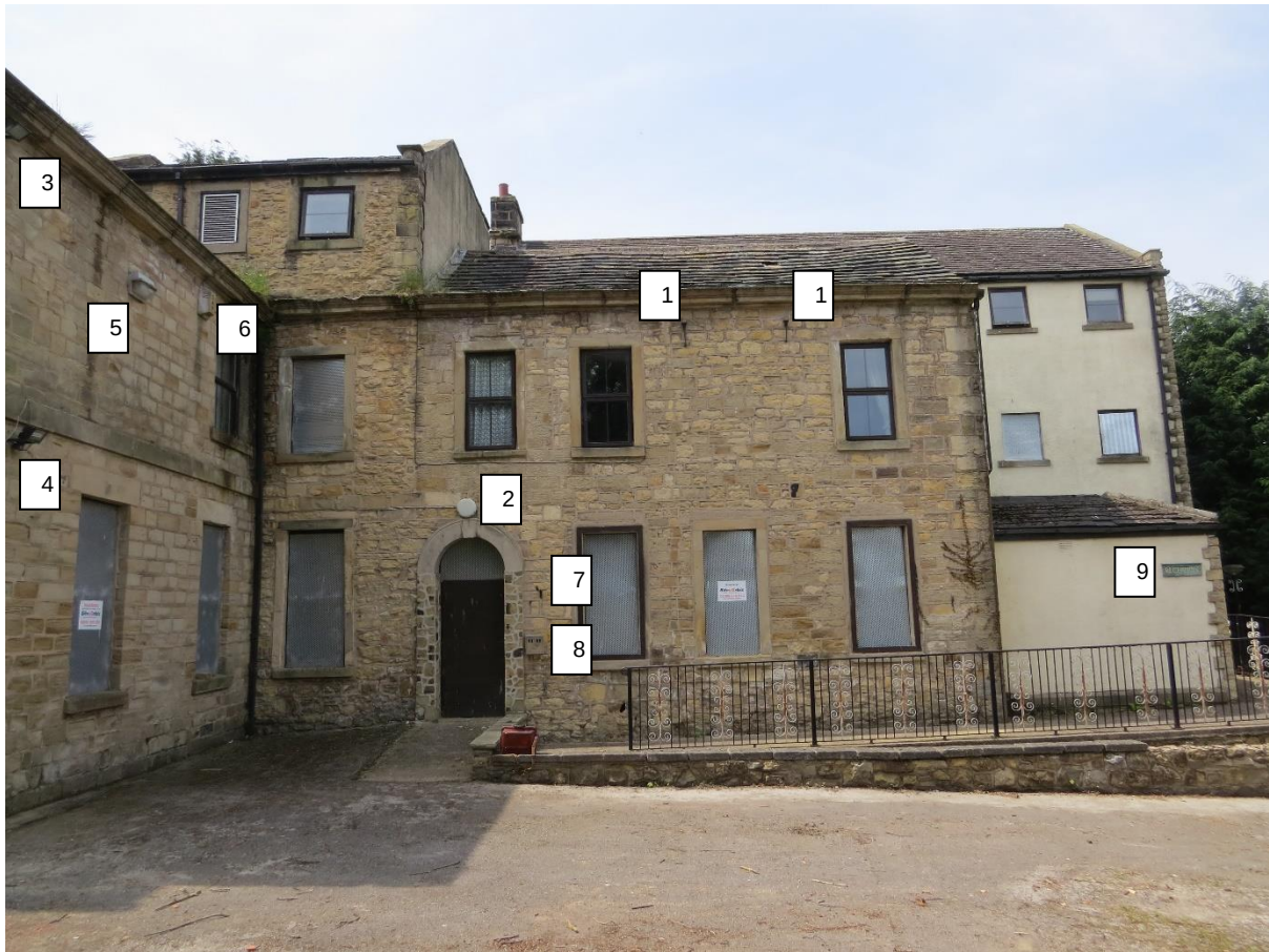
Fig 13 – East Elevation – removal of redundant fittings
