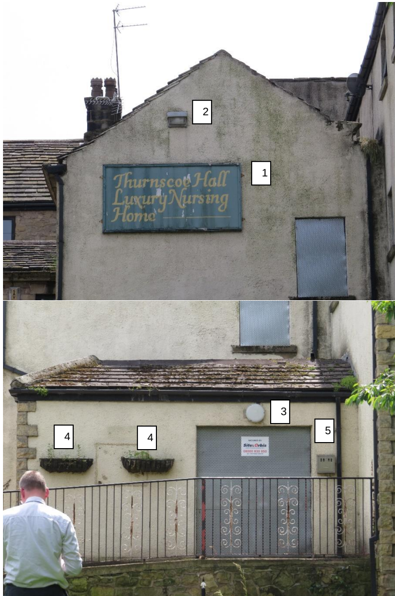
Figs 14 & 15 – North Elevation – removal of redundant fittings
