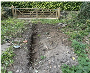
Inset: Root inspection trench
