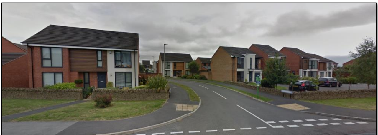
Newly built contemporary properties off Lee Lane
