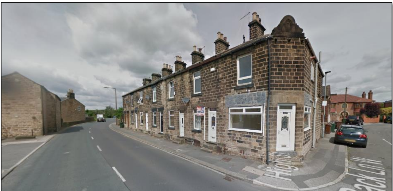
Existing stone properties on Lee Lane
