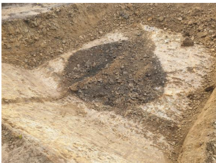
Photo 7 and 8: Mine entry F4 at surface (Top) and at rockhead (Bottom)
