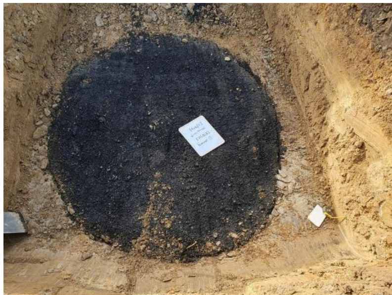
Photo 1 and 2: Mine Entry F1 at surface (Top) and at rockhead (Bottom)
