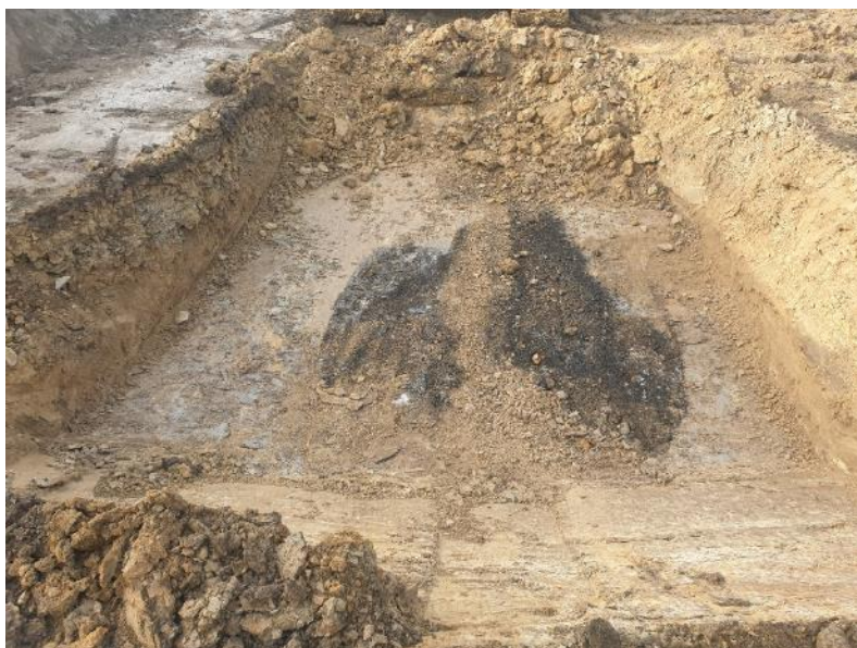
Photo 5 and 6: Mine entry F3 at surface (Top) and at rockhead (Bottom)
