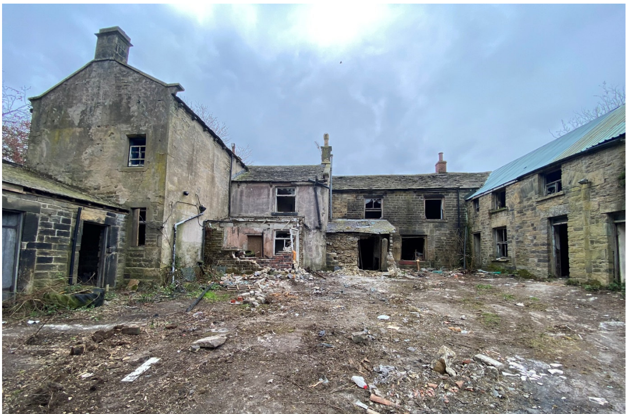
Photograph 2 – Cottages and outbuildings in the central area
