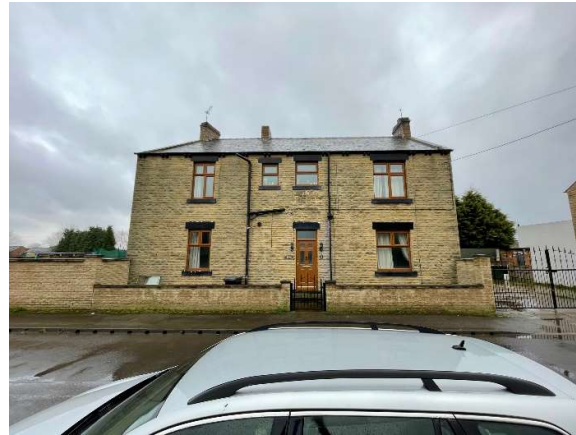
Overall existing front elevation.
