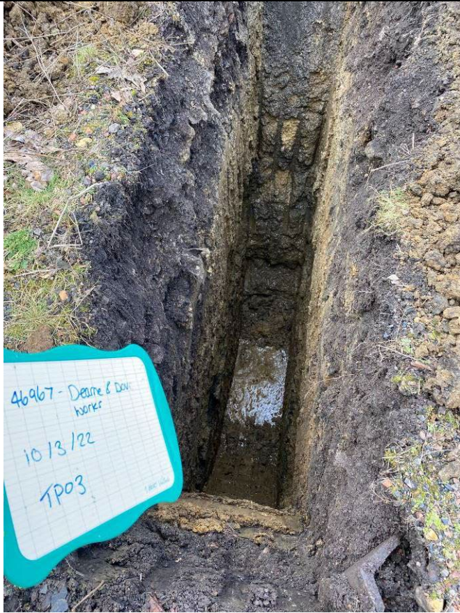
TP03 in the south west
