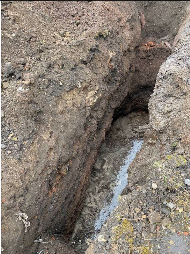
TP14 in the south west
