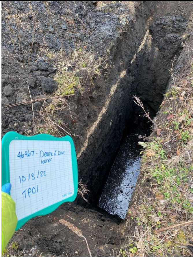
Trial Pit 01 in the south west corner
