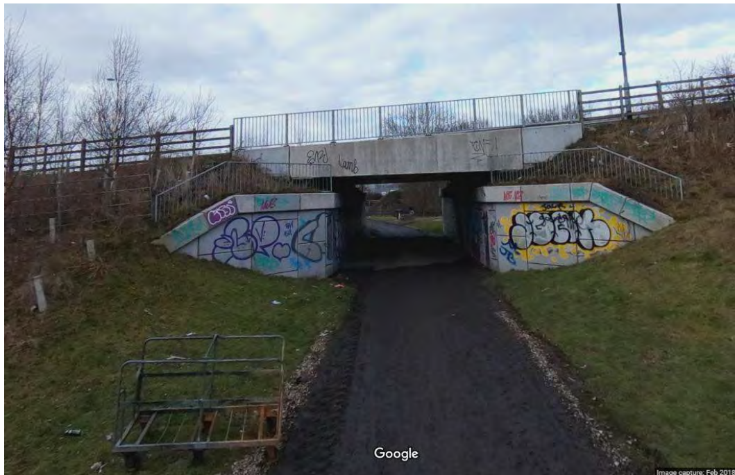
Figure 12: Old Tannery Road underpass (Source: Google Streetview 2021)
