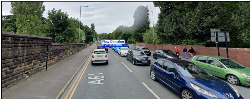
Figure 10: A61 Bridge walls looking west towards Barnsley (Source: Google Streetview 2021)
