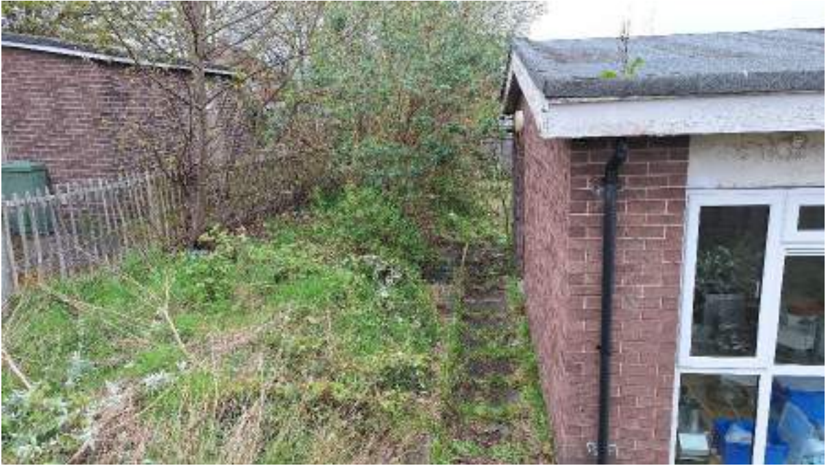
Plate 3: Cut slope between bungalow and sub-station
