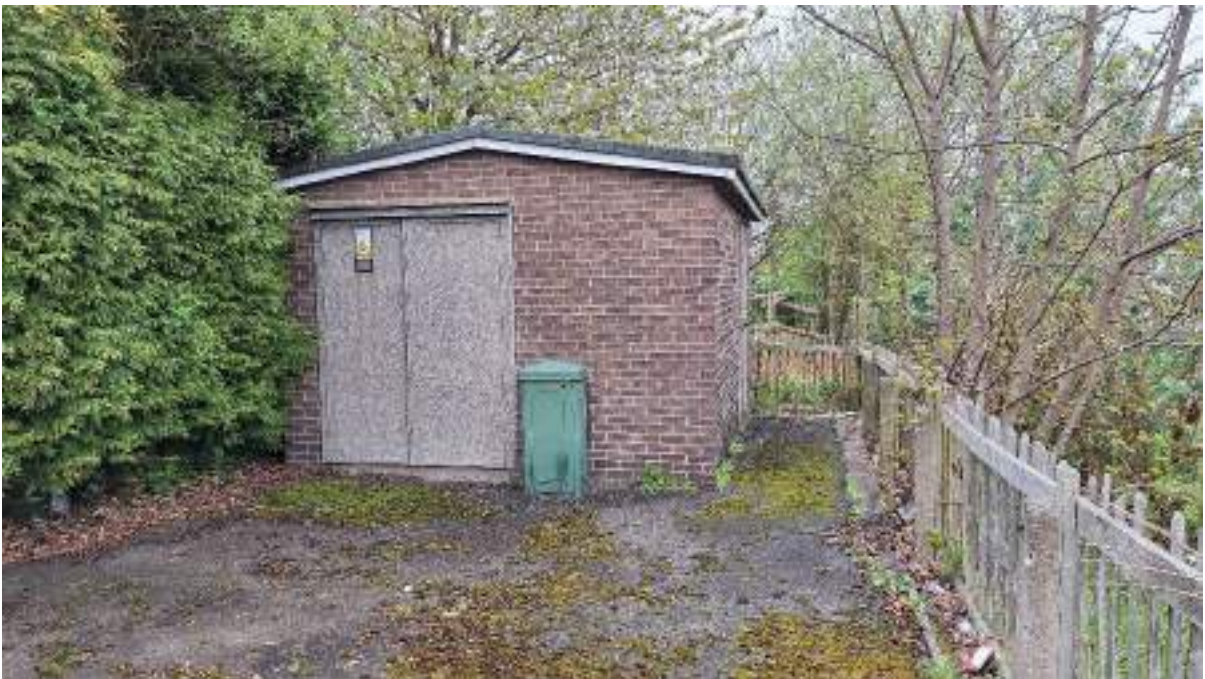
Plate 2: Electricity sub-station to west of site
