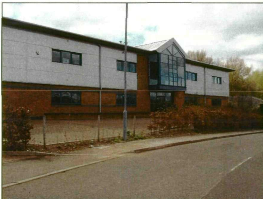
Photo No. 2 – Elevation showing view from Oakwell View
