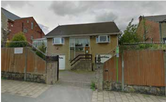
Front of the existing dwelling
