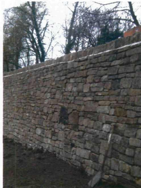
Random rubble uncoarsed in facework to concrete, with recessed mortar
