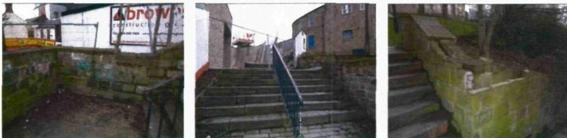
Photographs of existing scheme
