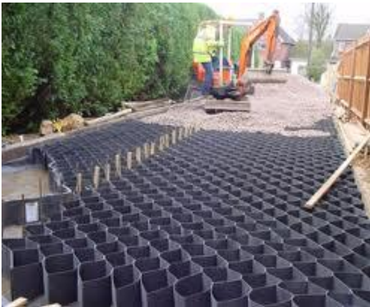
Figure 2. Example Cellular Confinement System (CCS)
