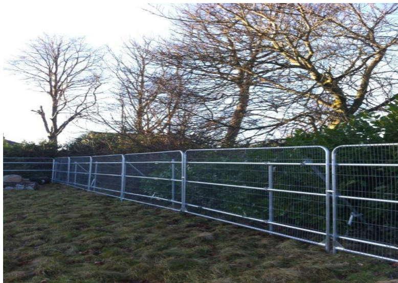
Photograph 1. Example of BS5837:2012 Protective Fencing
