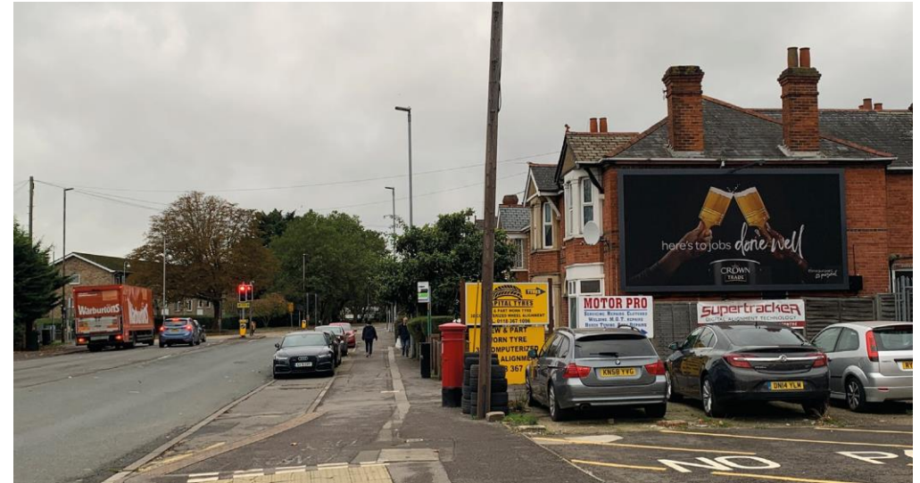
AFTER: Gable mounted 48-sheet digital advertising display.
