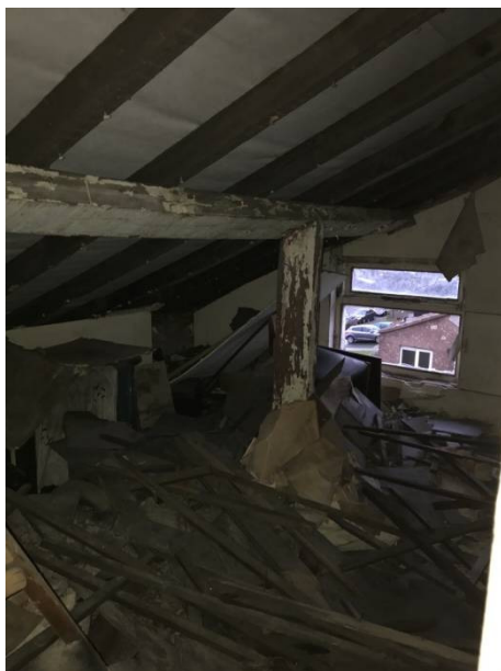
Above: The existing Roof space Right: Ground floor former bar area
