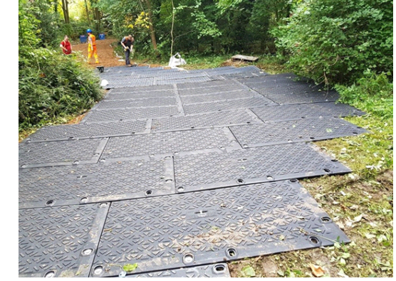
Inset 3: Interlinked ground protection boards
