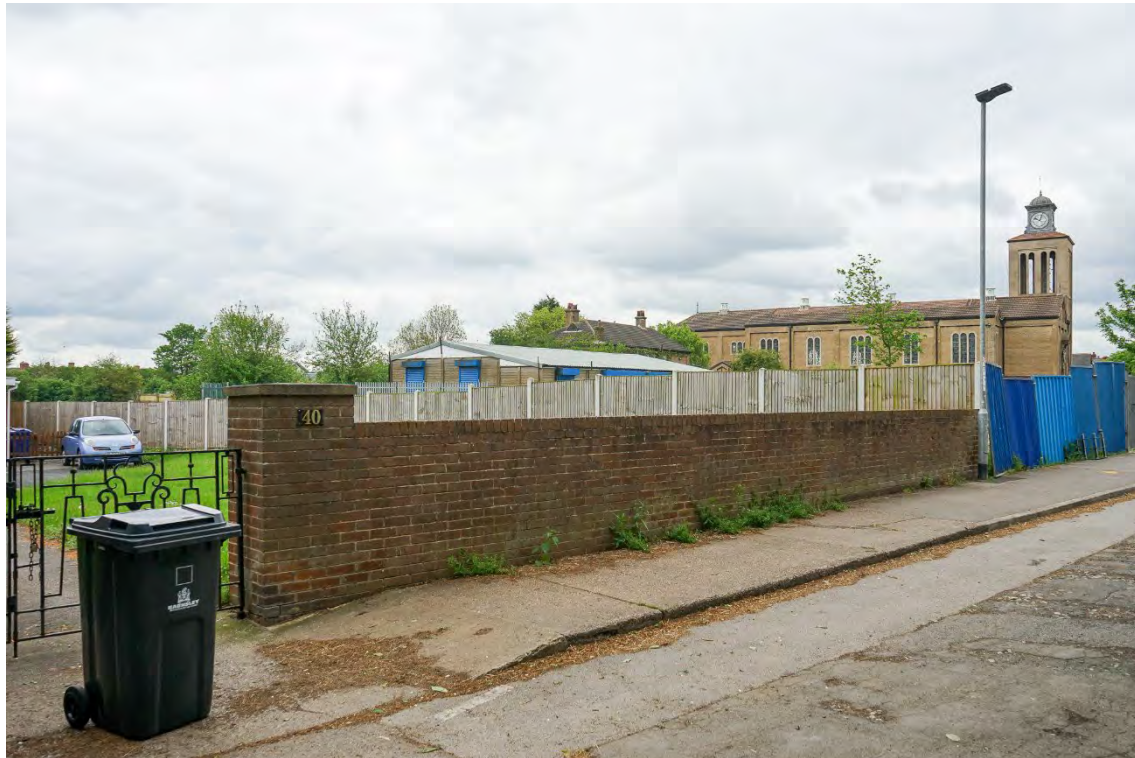
Photo 11: View to the Church of St John and St Mary Magdalene from Lockwood Road, with the wall to No.40 Lockwood Road, fencing, and the scout hut in the foreground
