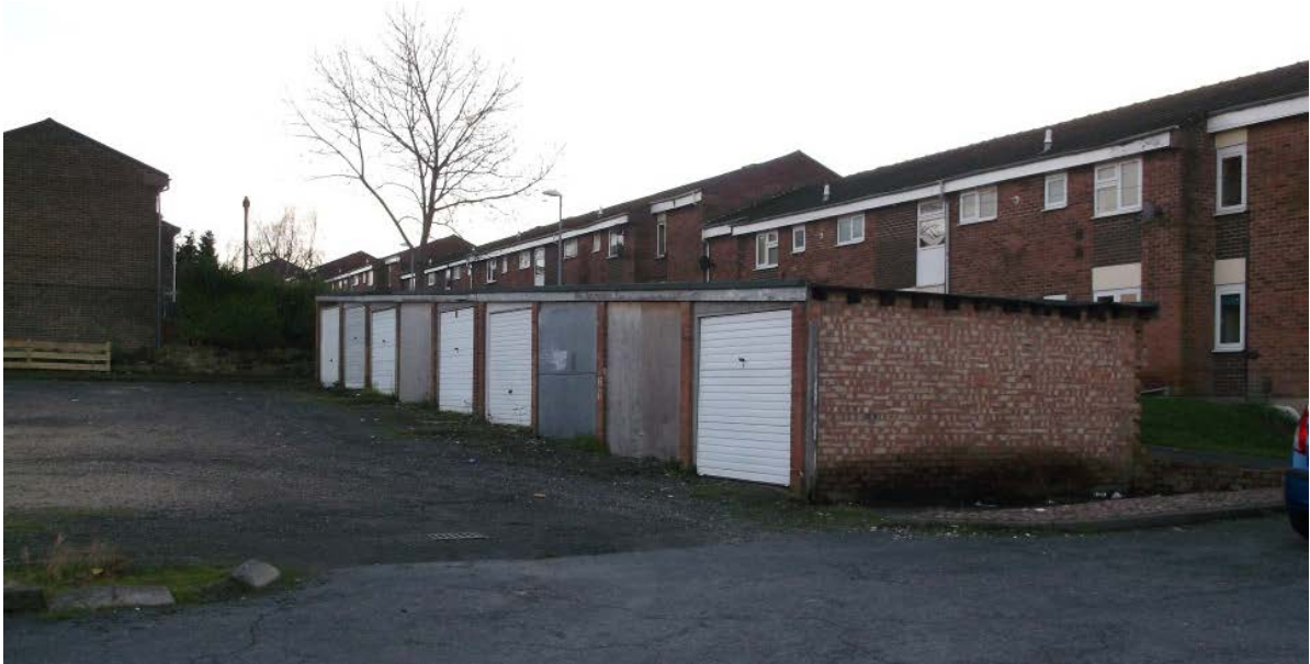
View of redundant / boarded garages located on site
