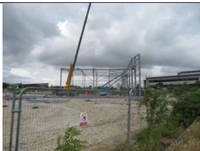
Photo 1: Active Construction to the east of Unit 6
