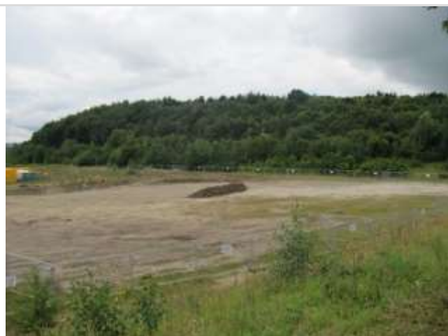
Photo 3: Cleared ground at the north of the site
