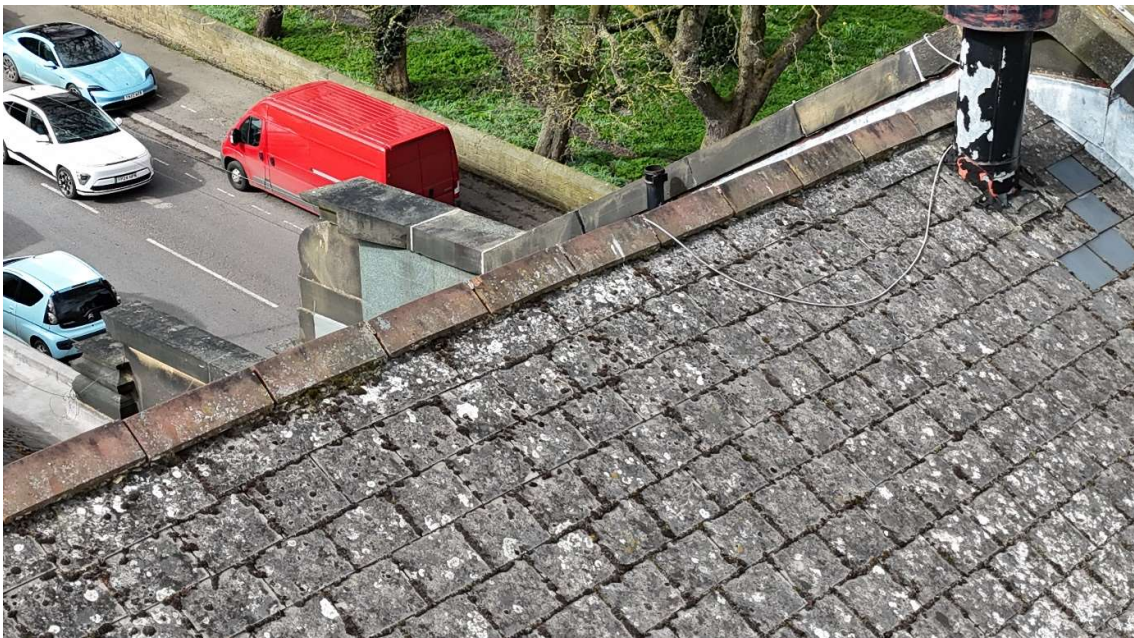
Close view of pitched roof covering Inc. ridge tiles
