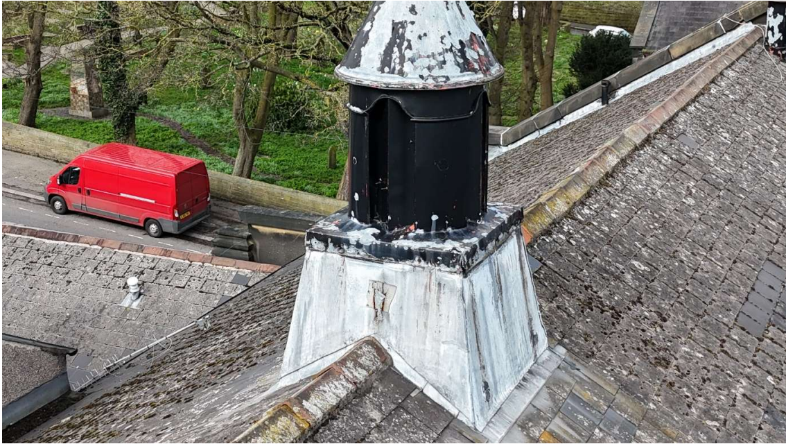
Typical roof cowl to be removed
