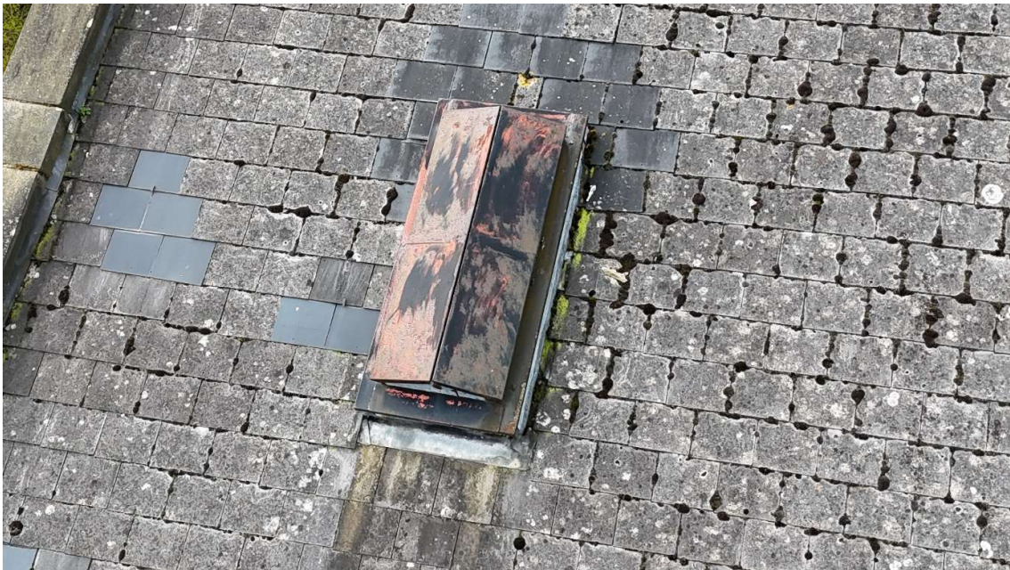
Typical roof vent to be removed
