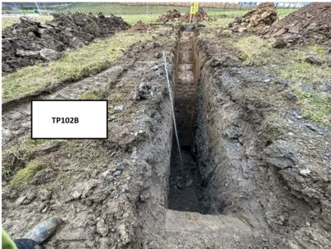
Figure 4: Photograph of TP-102b showing a vertical face into the opencast material.
