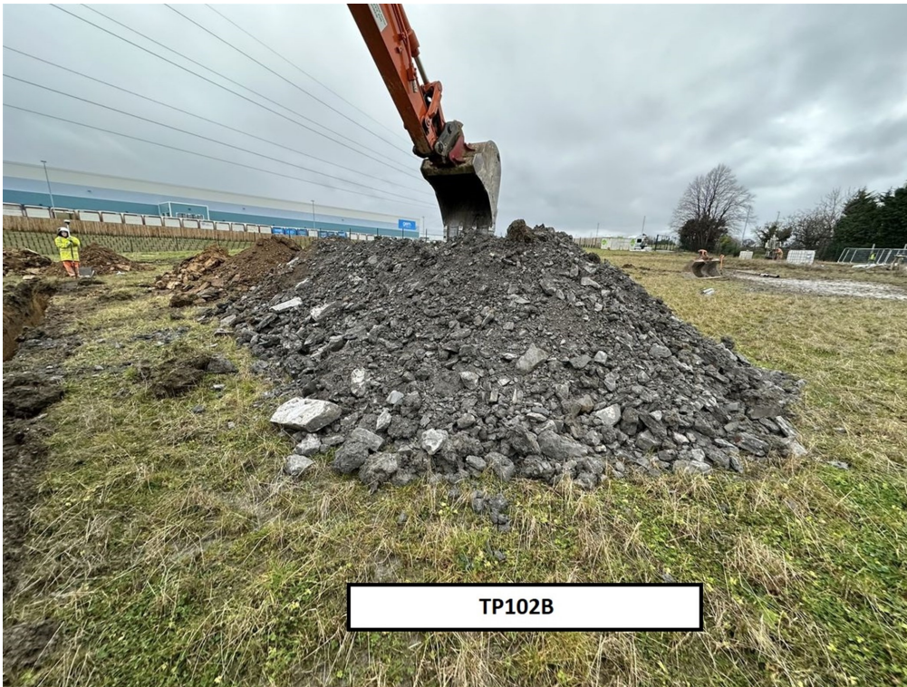
Photograph 15: Trial pit TP102B. Trial pit arisings (2). View from east to west.
