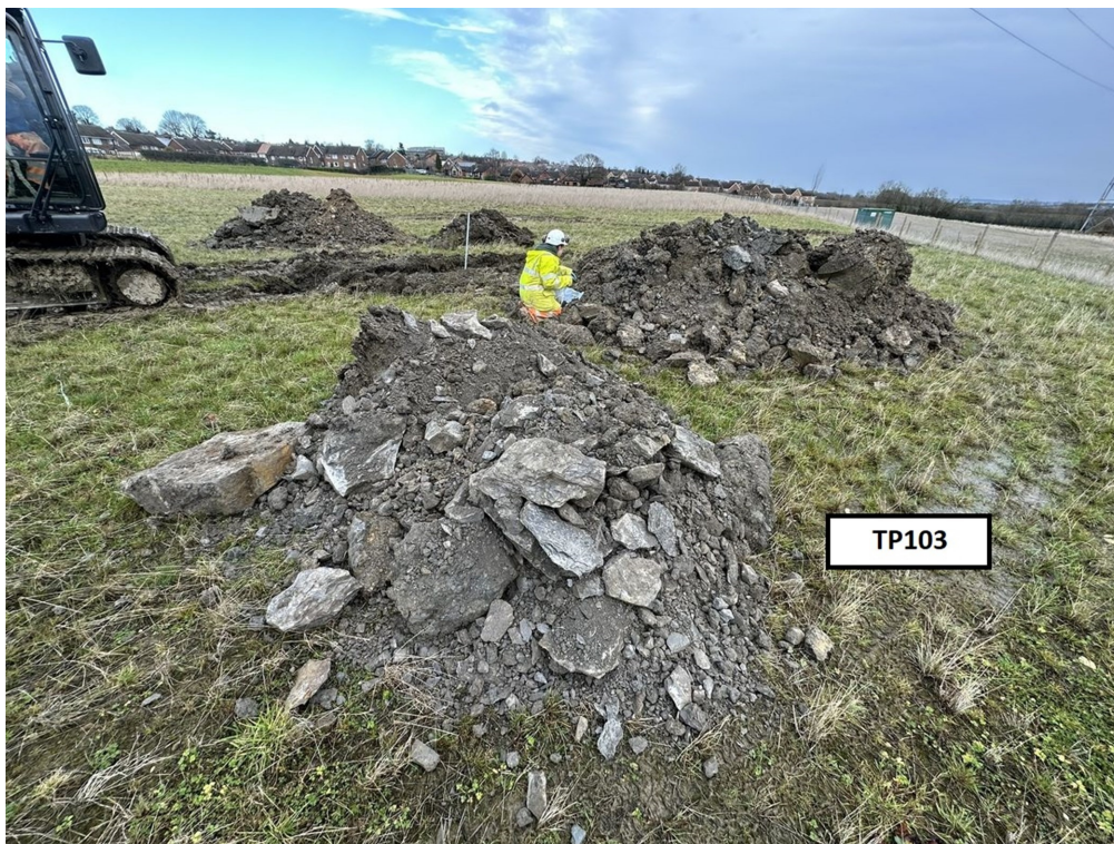
Photograph 22: Trial pit TP103. Trial pit arisings (3). View from south west to north east.
