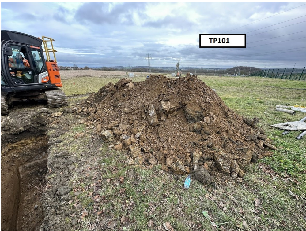
Photograph 04: Trial pit TP101. Trial pit arisings (1). View from north west to south east.
