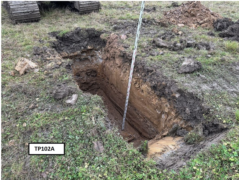
Photograph 08: Trial pit TP102A. Northern and eastern sides of trial pit. View from south west to north east.
