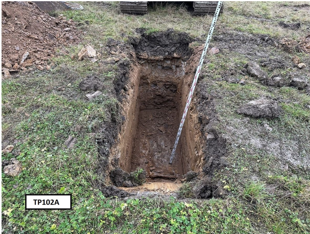
Photograph 06: Trial pit TP102A. View of trial pit from south west to north east.
