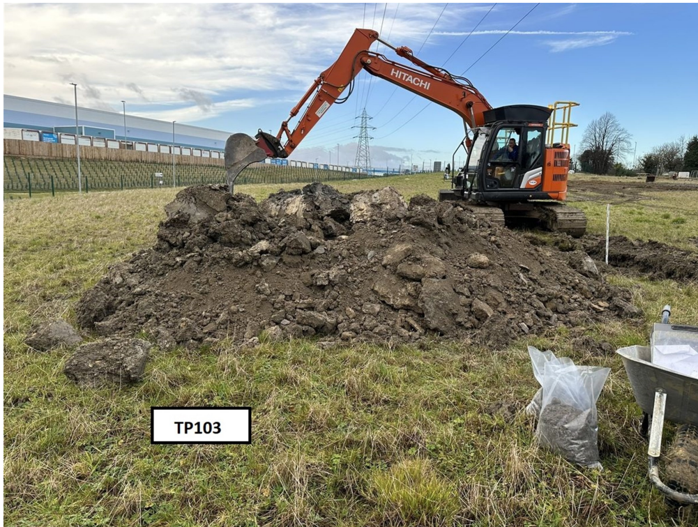
Photograph 21: Trial pit TP103. Trial pit arisings (2). View from east to west.
