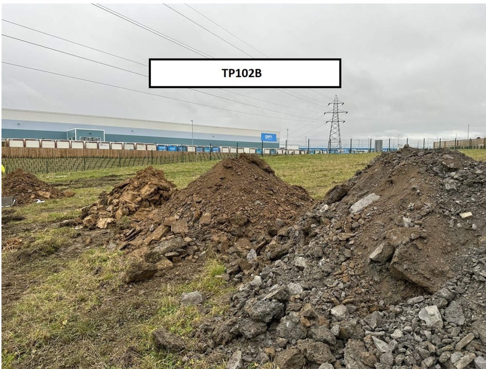
Photograph 16: Trial pit TP102B. Trial pit arisings (3). View from east to west.
