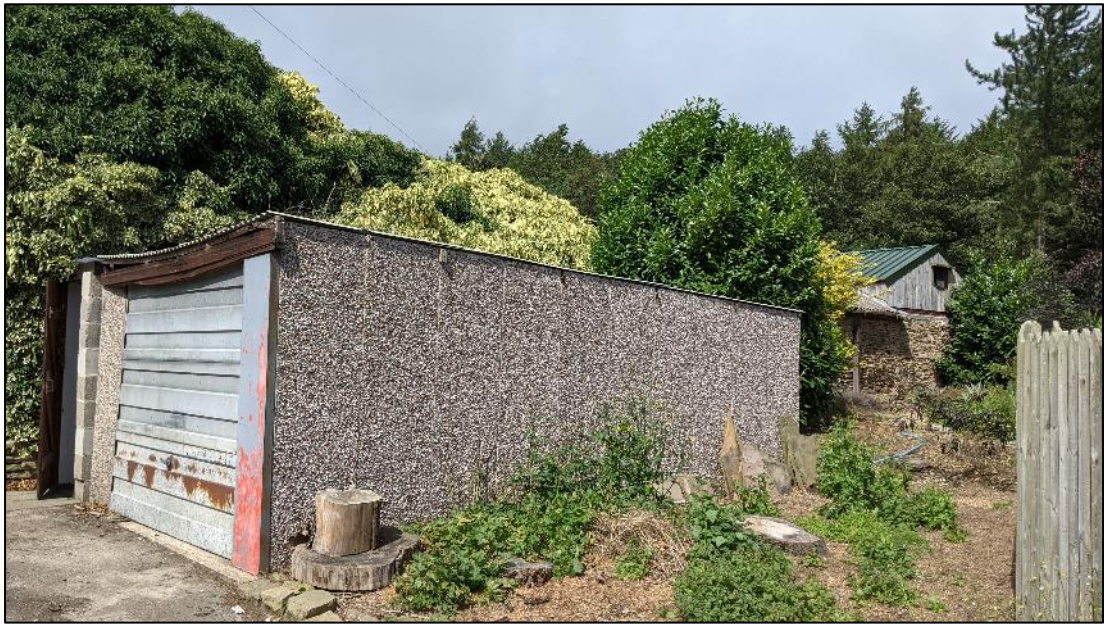
Potential roost features on building exterior – Outbuilding
