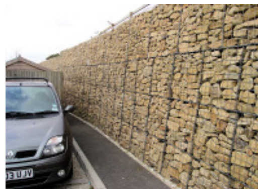
Stone Filled Gabion Baskets
