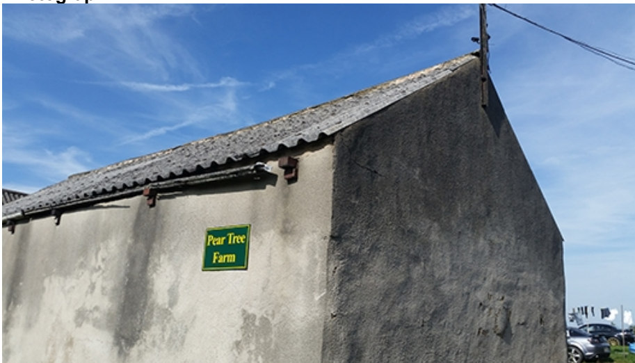
Building A4, south-east gable end
