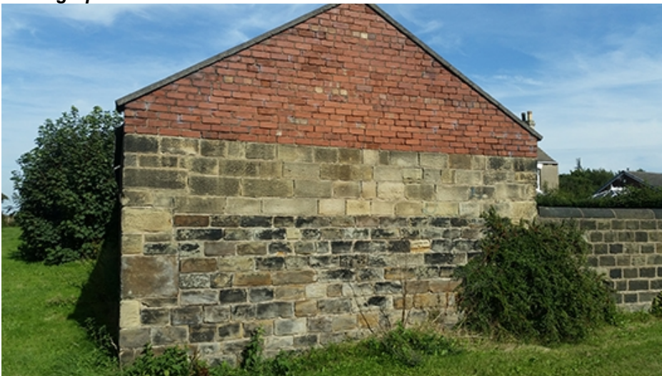
Building A1, north-west parapet gable
