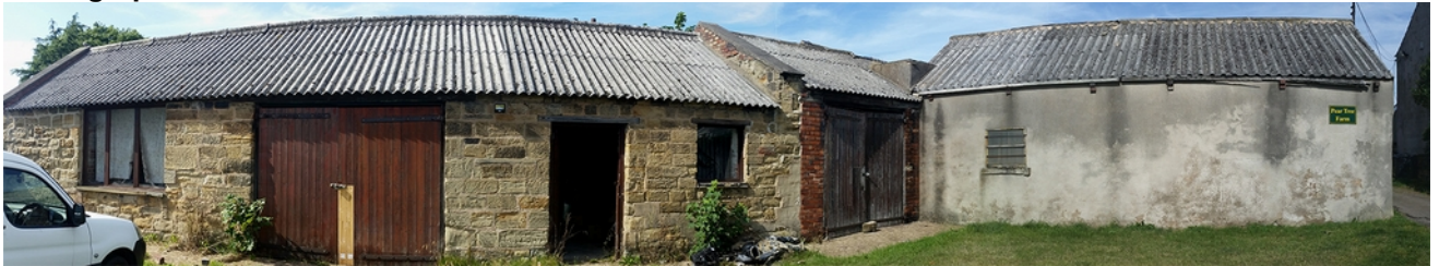
Building A1, A2, A3 and A4, south elevation
