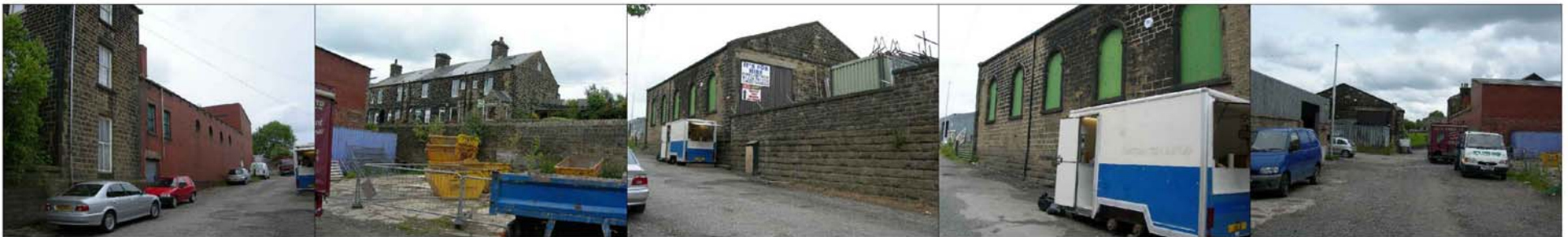
Looking up and down proposed access road
