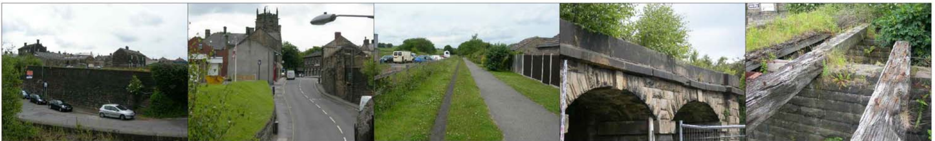
Looking from top of Drops to new roundabout
