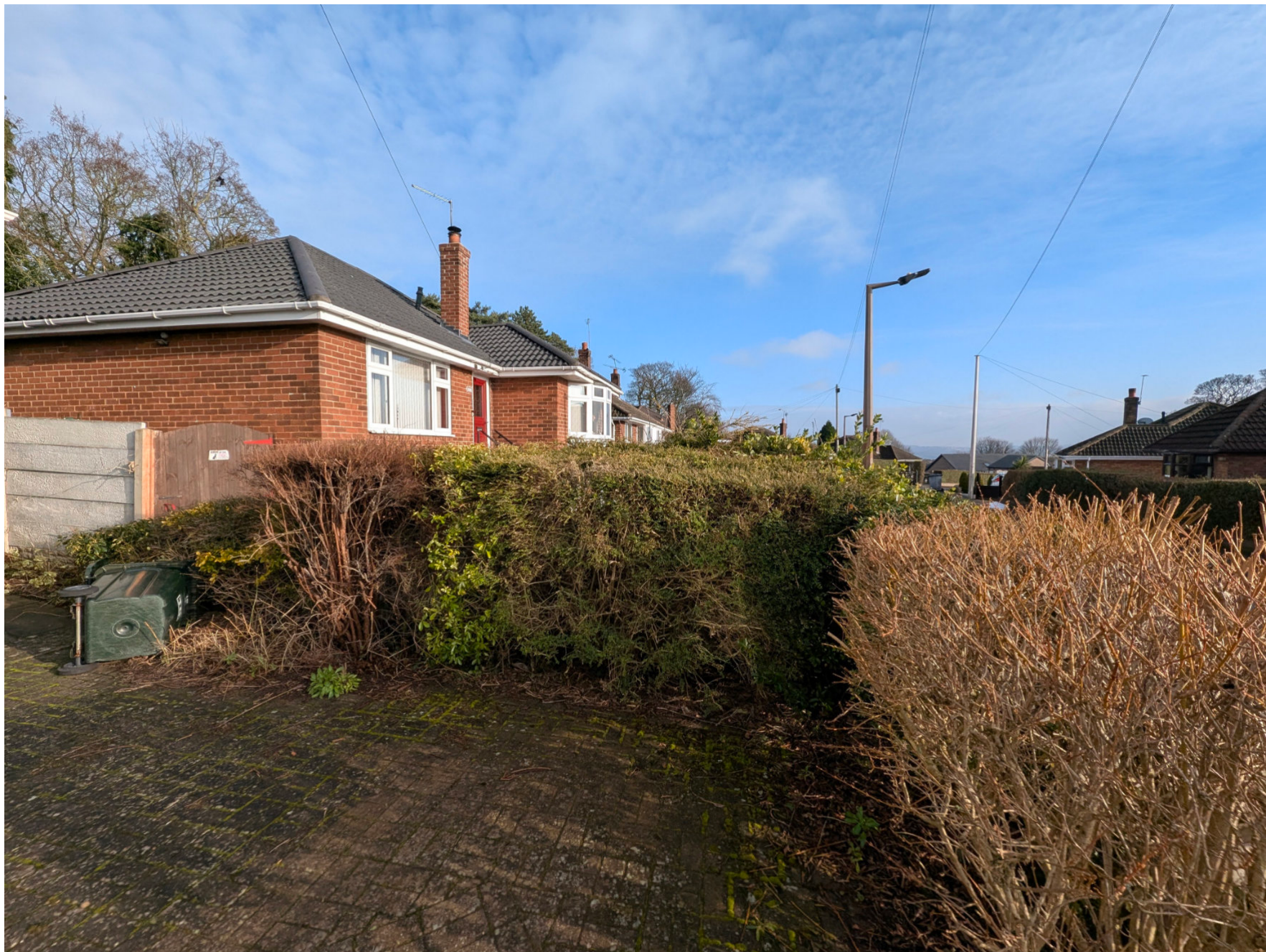
2407 - 10 Wentworth Way, Dodworth, S75 3RA Neighbouring properties to East
