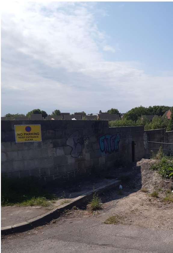
Existing blockwork wall to be demolished to allow for new road access to site
