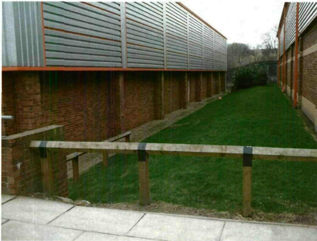
View of Existing Side Elevation looking towards rear.
