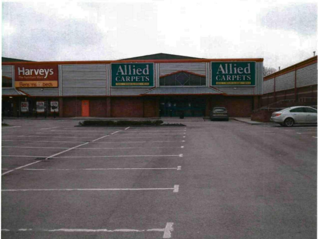
View of Existing Front Elevation from the customer car park.
