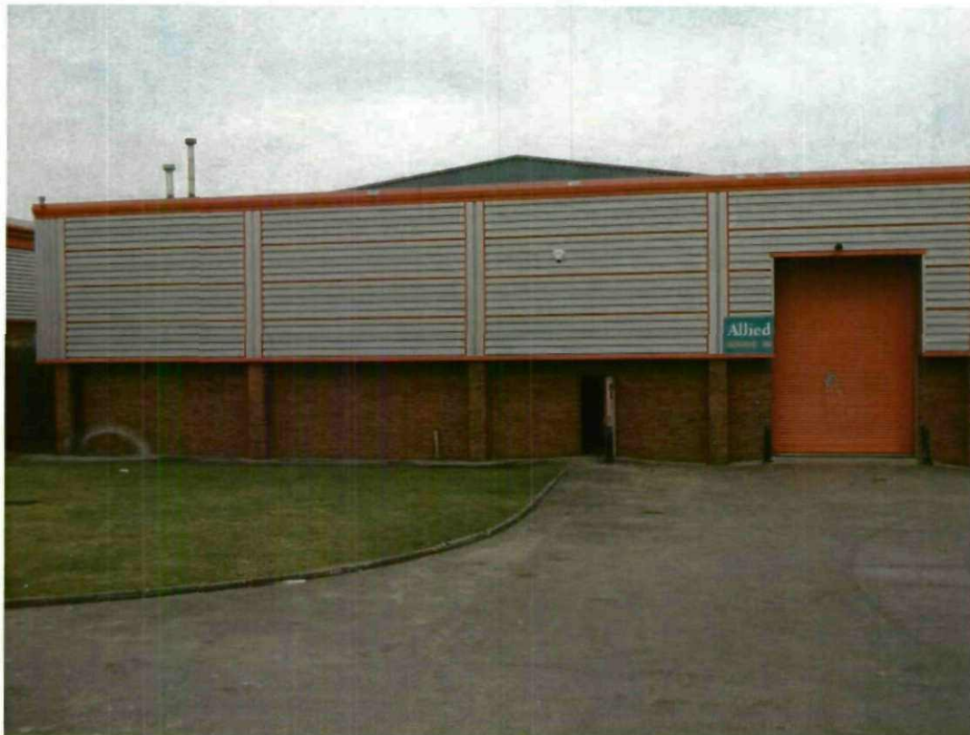
View of Existing Rear Elevation.
