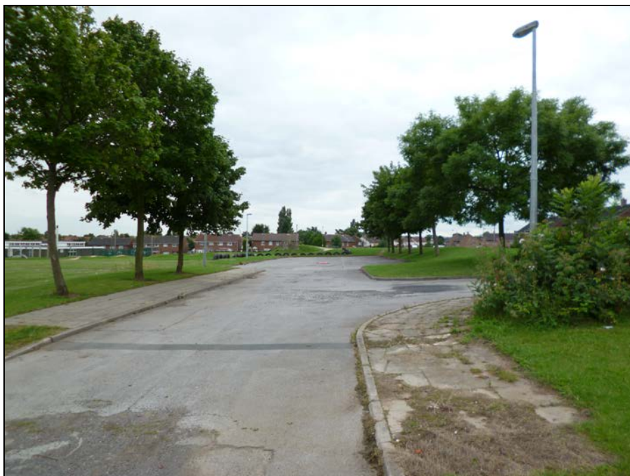
Plate 5: View looking south along the western boundary. .
