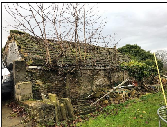
Figure 3: The northern elevation of the building.
