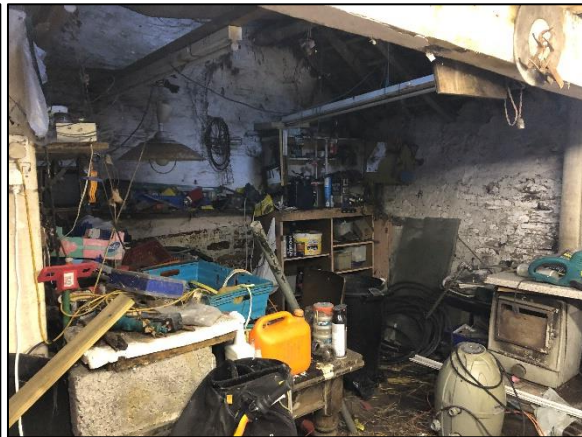
Figure 6: The interior of the workshop/storage area.
