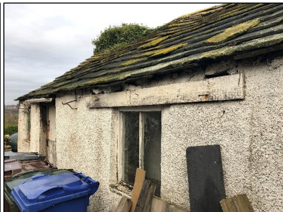
Figure 9: Rendered areas to the south of the building.
