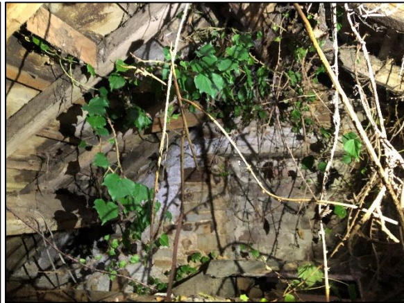
Figure 14: The loft space to the west of the building.
