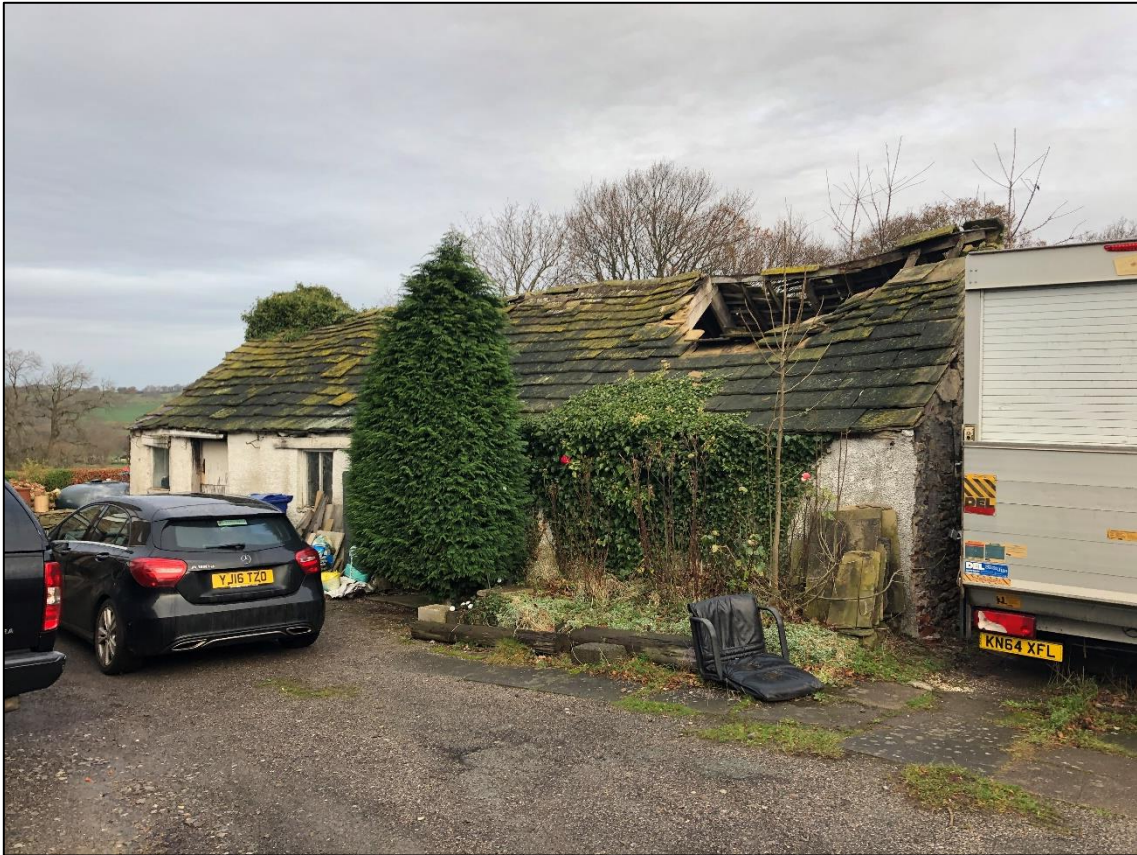
Figure 2: The southern elevation of the building.
