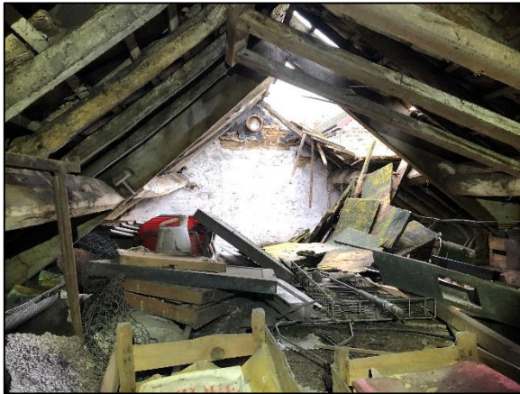
Figure 13: Looking along the interior of the building.
