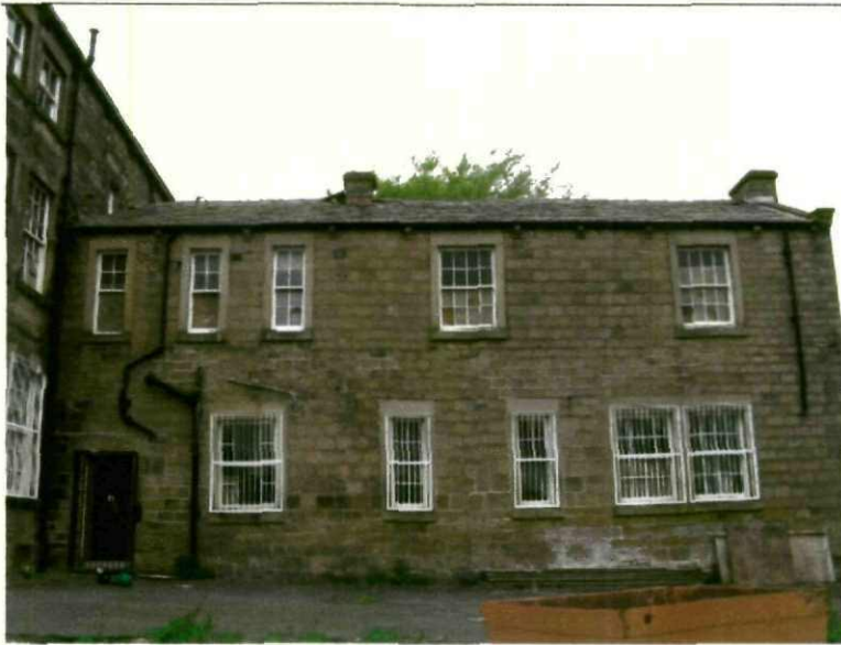
Figure 3 View of extension attached at eastern elevation.
