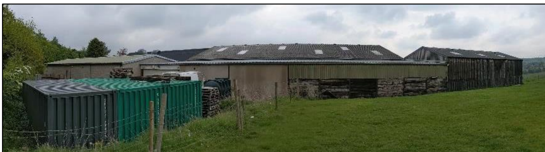
Plate 3. Northwest side of building complex with BS12 on left of image, BS2 in centre and BS11 on right
