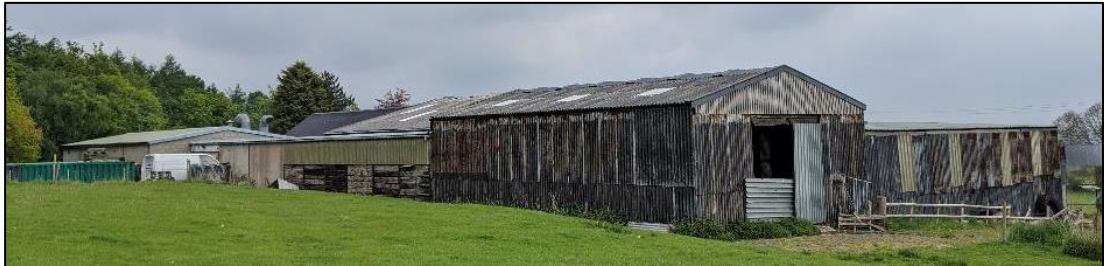
Plate 10. Building Sections 12 & 2 on left of image with BS11 in centre and BS10 on right
