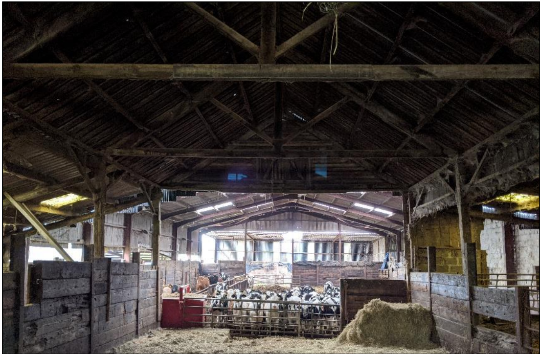
Plate 4. Interior of BS3
