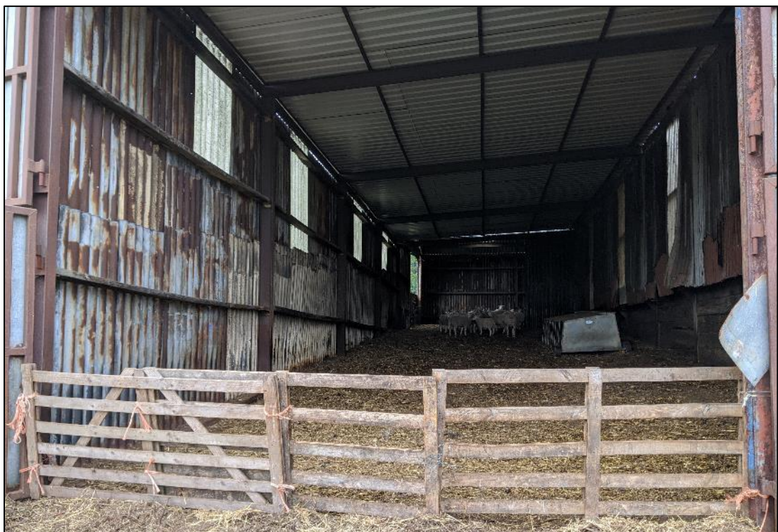
Plate 9. Interior of BS10
