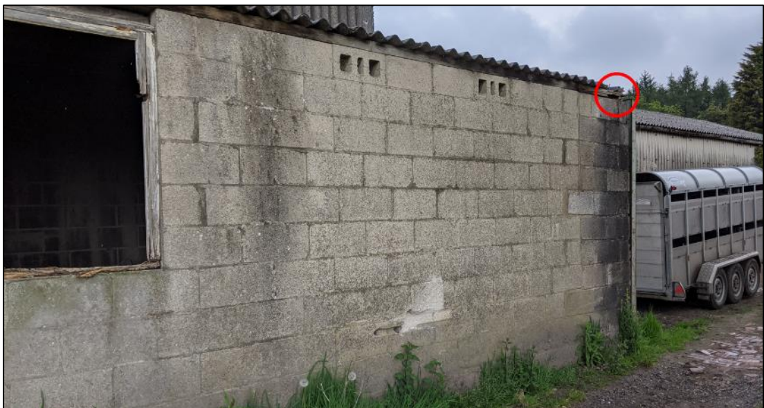
Plate 8. Southeast elevation of BS7, with house sparrow nest location indicated by red circle
