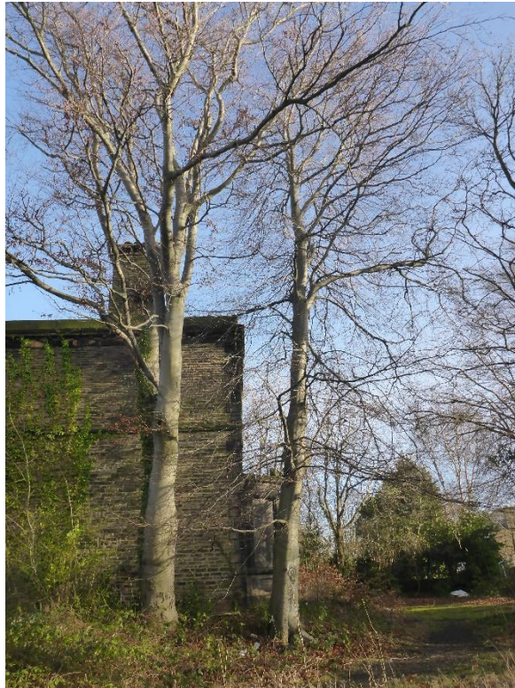
Photo 8: T14 (right) and T15 (left), situated in very close proximity to the existing building.
