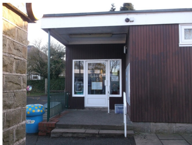
View of West Riding Block to be demolished as part of the development
