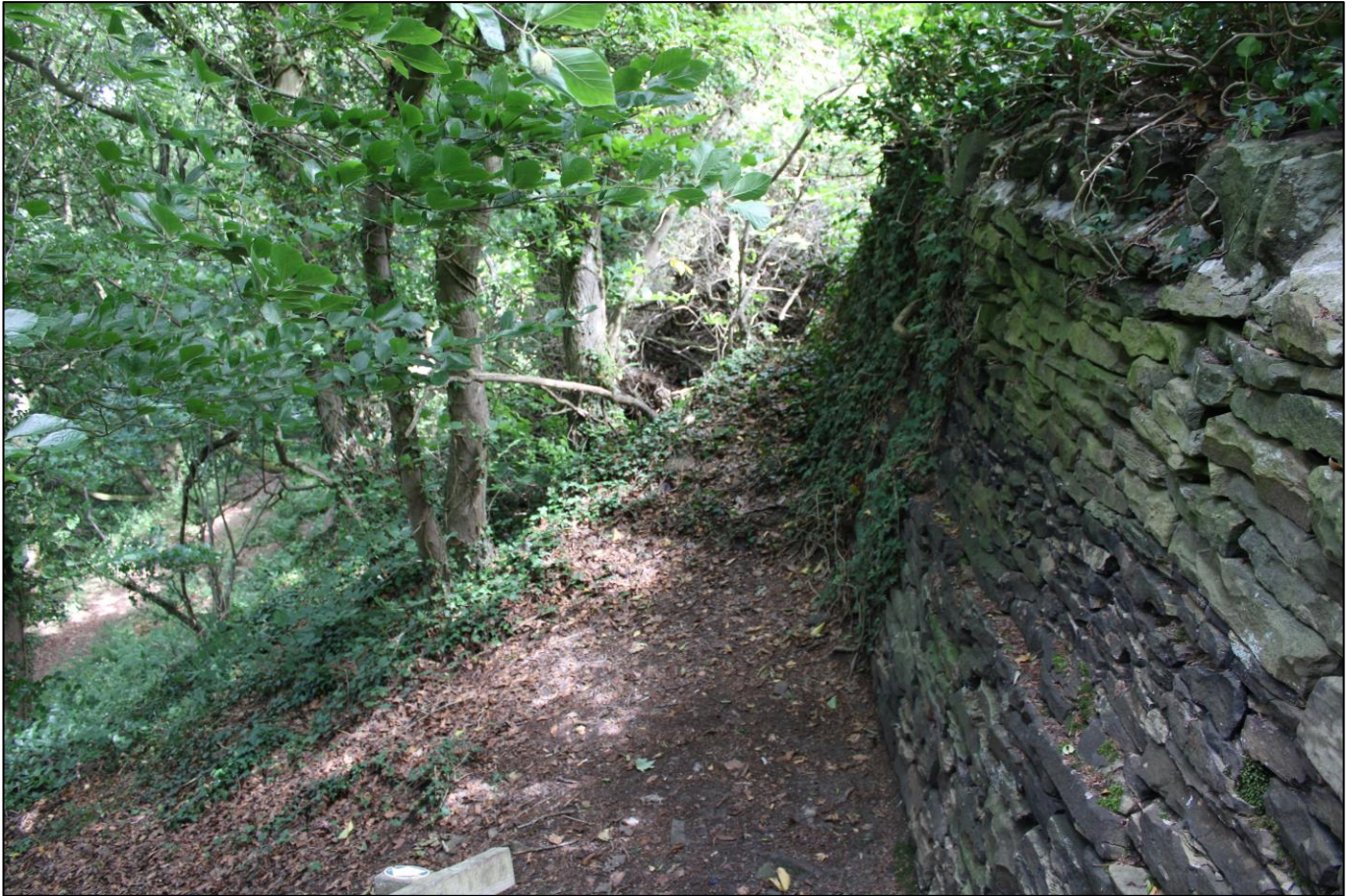
Photo 2: view of the retaining wall and steep bank below the northwest side of Litherop Road.
