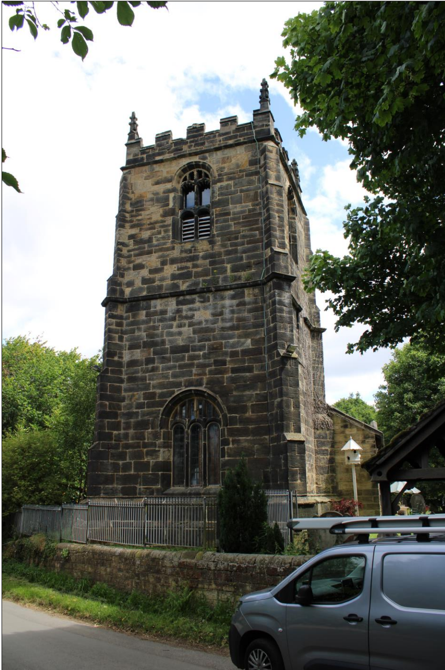
Photo 7: The west face of the tower, looking east from Church Lane.
