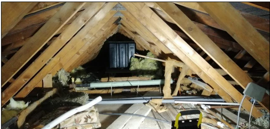
Plate 11. Roof-space of dwelling
