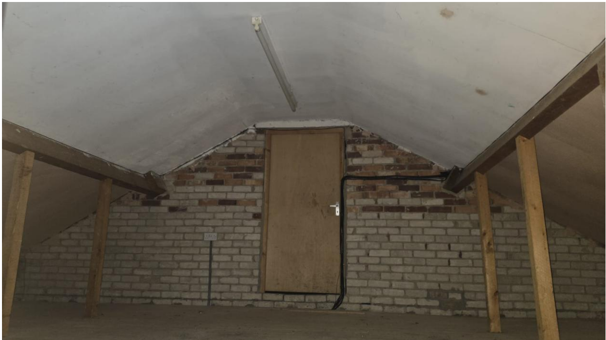
Photograph 4: Inside garage roof void
