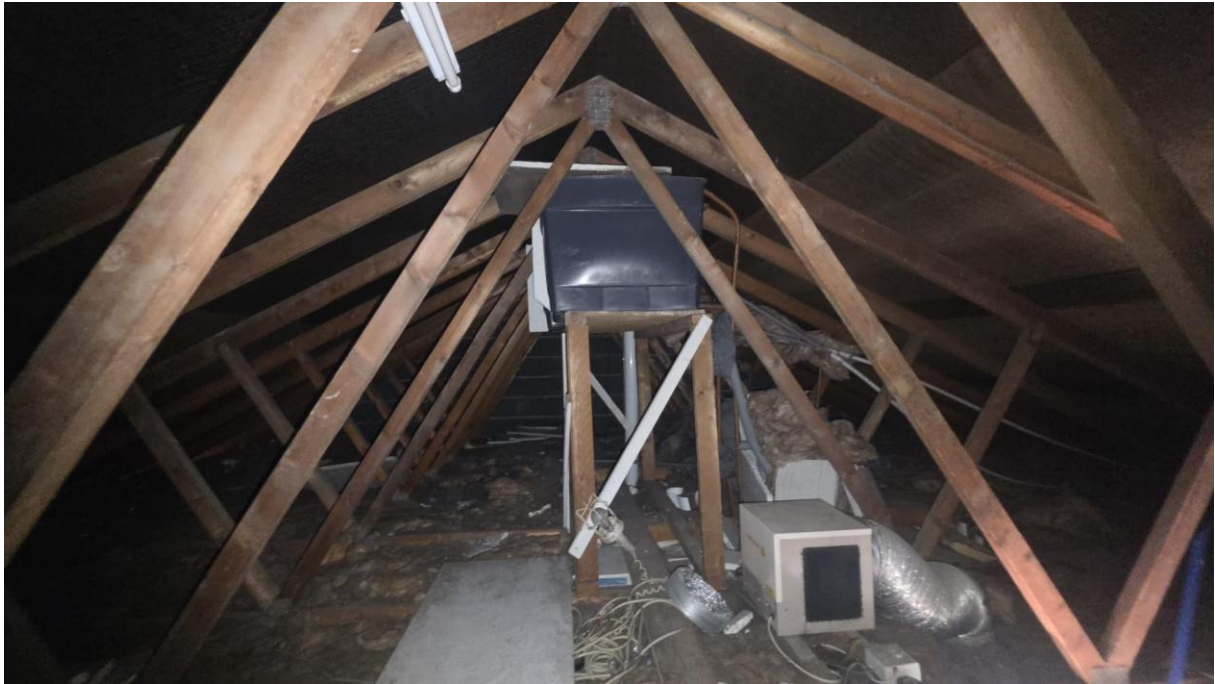
Photograph 5: Inside main roof void
