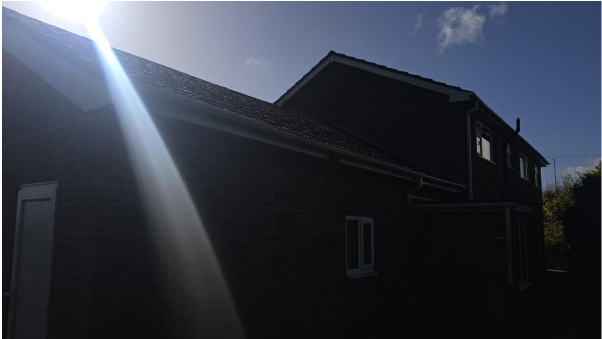
Photograph 3: Rear of building.
